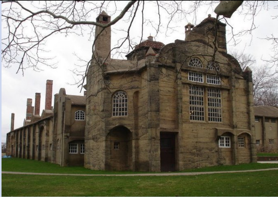
The Tile Works of Bucks County, Doylestown Township
